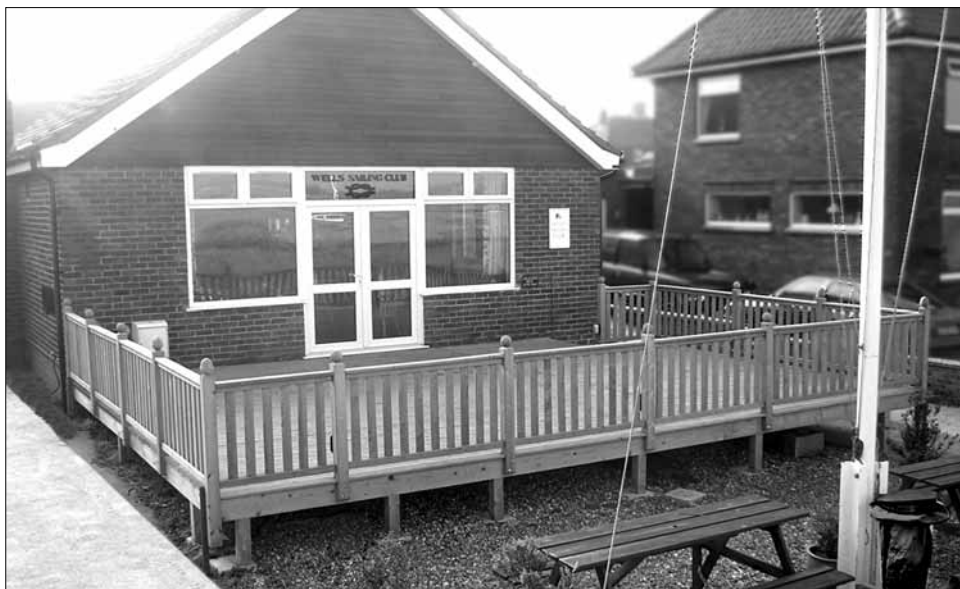
The newly-extended decking
